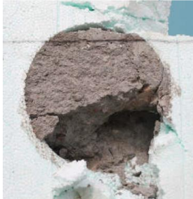
Anchor installed on a skew
